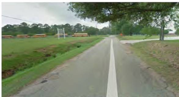
The project consisted of rehabilitating a 2,700-ft section of the most traveled local roadway in the Parish. Bains Road is the sole local roadway providing access to West Feliciana public schools.
