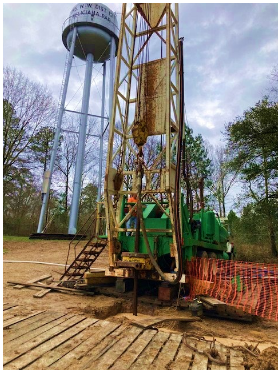
Drilling Weyanoke Well No. 2
